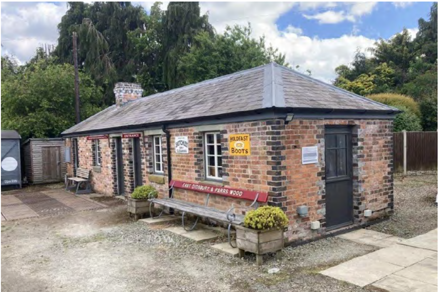
In contrast to the derelict condition shown on the previous page, the weighbridge building at Bishop's Castle has been fully restored and is now the Bishop's Castle Railway Museum.
