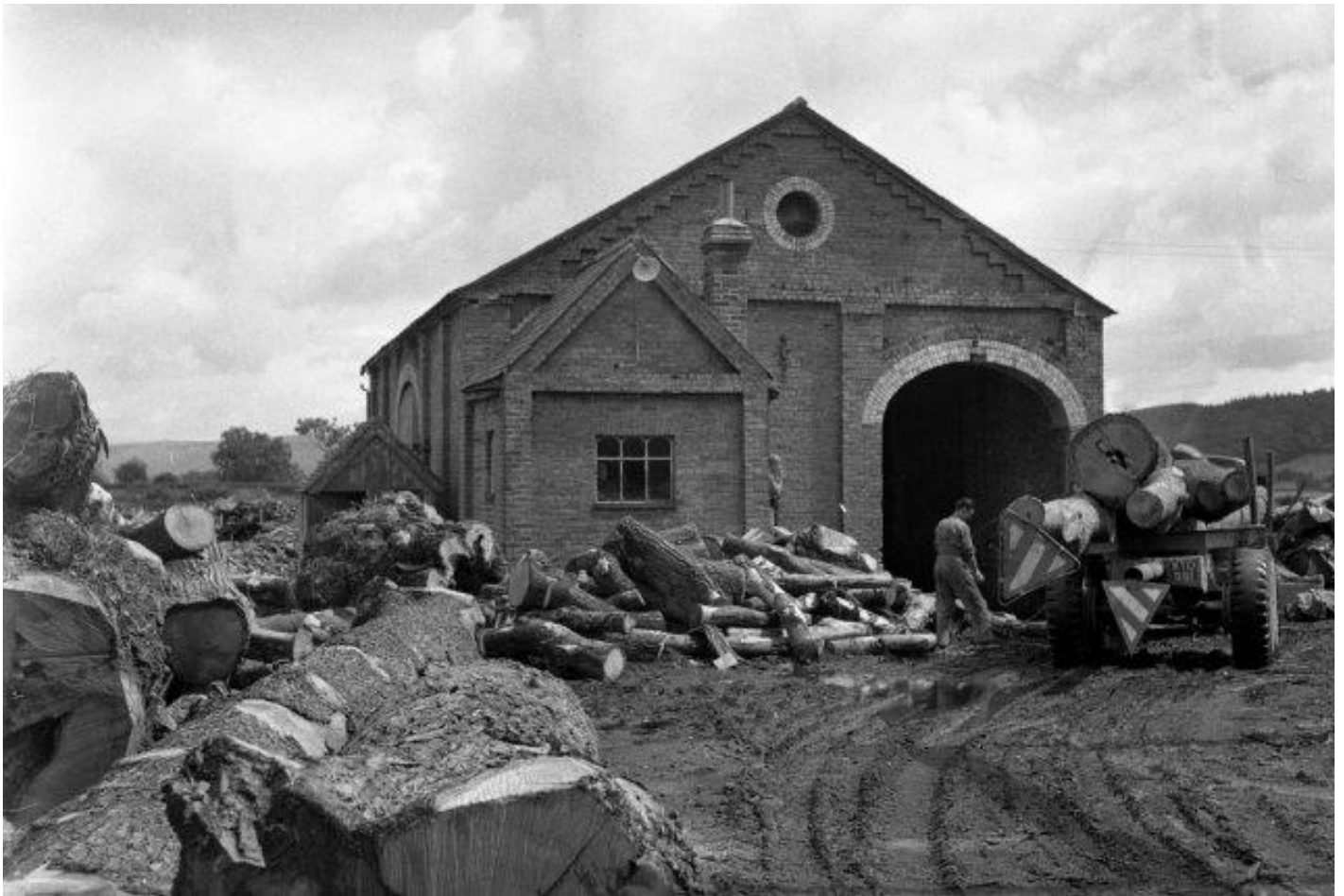
The goods shed as it was on 4th August 1966.
