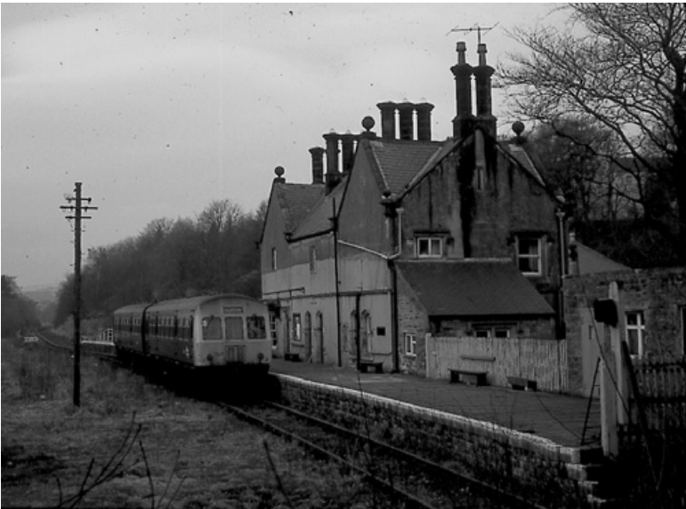
The overall roof and loco shed have long since disappeared but the station building has survived at the terminus of the Alston branch, as a DMU waits to return to the junction on the soon to be closed branch from Haltwhistle. 21 February 1976.
