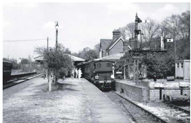
Horsted Keynes also exhibited an air of near neglect back on 9th May 1970 when a handful of passengers waited to board a train for Sheffield Park behind 27.
