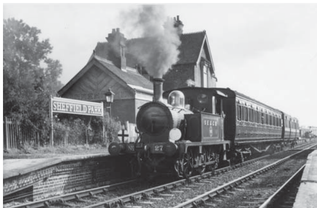
SECR 27 prepares to depart from Sheffield Park on 21st September 1968 when the station looked very under developed compared to today.
