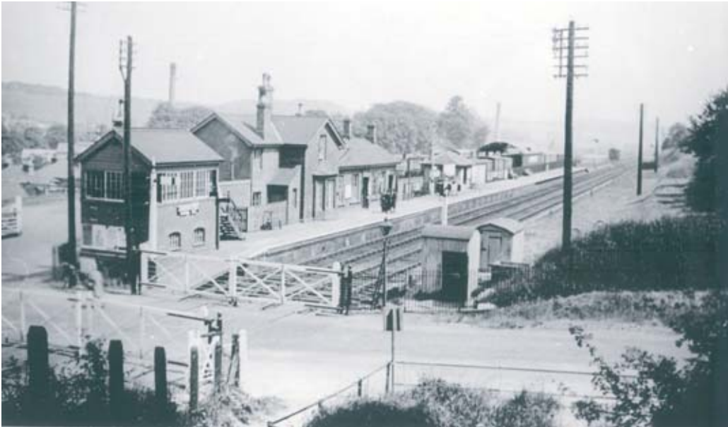
Taken in 1932 from the same viewpoint as the photograph opposite with the station house extended and the waiting veranda now filled in. At the far end of the platform there is a corrugated iron goods shed with Loudwater in large lettering on the side.
