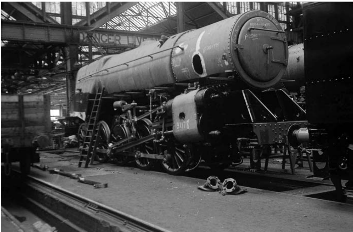
British Railway Standard 9F 2-10-0 92178 approaching completion inside the A Shop at Swindon in the summer of 1957. This was the first of the final batch built at Swindon culminating with 92220 Evening Star in March 1960.
