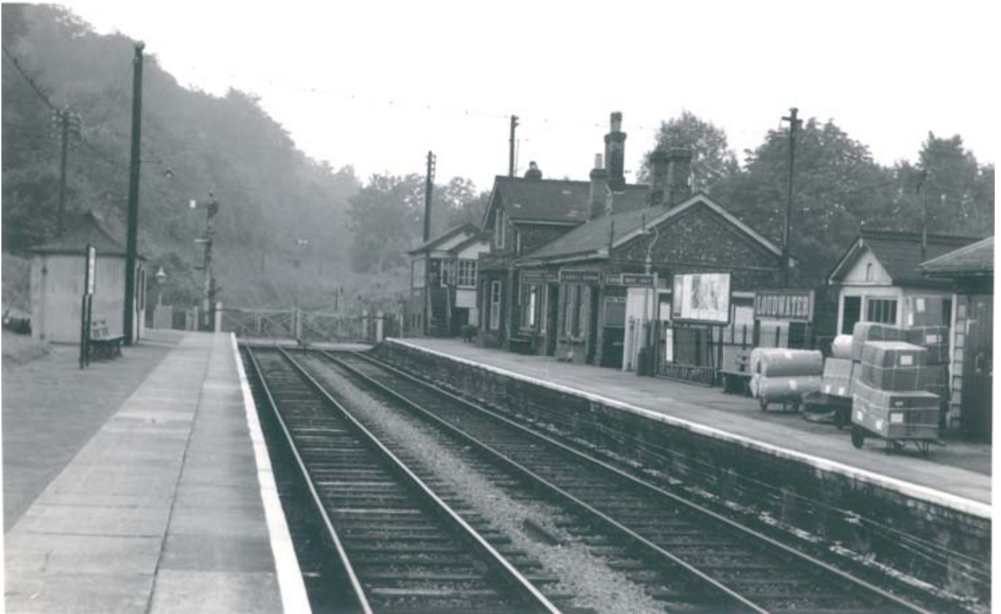
Looking towards High Wycombe circa 1959 with two signal posts visible and token apparatus. There was a trap point before the line curved round to the right. The nameboard in front of the pagoda waiting room pronounced 'Loudwater' home of Fords famous blotting paper.
